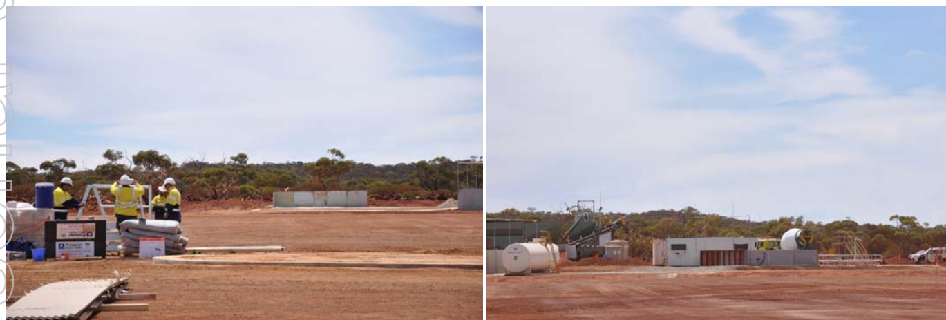
Karara site construction work and installation of the concrete batch plant
