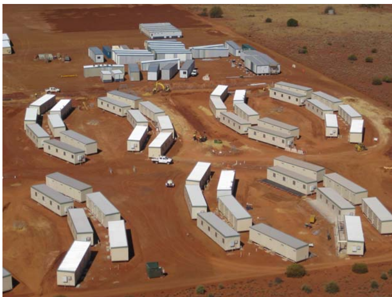
Aerial view of the Karara Village construction
