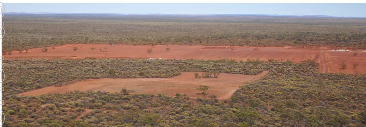
The view of Karara Ridge from the plant site (top) and the cleared site for the Karara magnetite processing plant (bottom).
