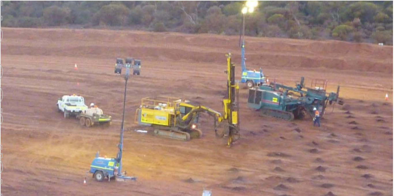
Drill and blast operations
